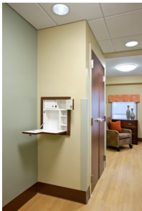
A nurse server (i.e., a lockable cabinet at the entry to a resident’s bedroom) provides easy access to meds and supplies, allowing the professional caregivers to stay engaged with the resident rather than off running errands.
