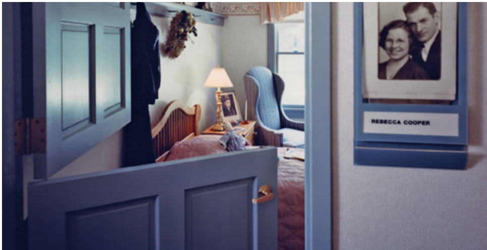
Dutch doors allow visual connectivity while limiting physical access into resident bedrooms.
